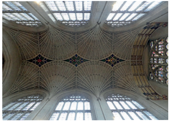
Fan-vaulted ceiling at the eastern end of Bath Abbey created in the 1500s by Henry VII's master masons. Photo: Diane Davies
